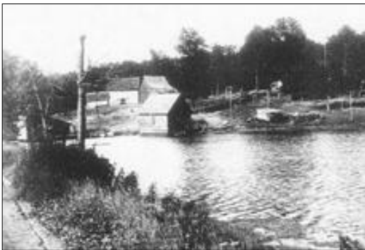
Spring Brook Farm. Site of dam where Aaron Dahlberg first generated electricity.
