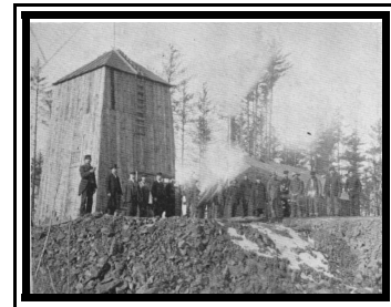
Figure 9. The Chippewa Mine, 1900. Located on the Middle River near the end of Twenty-Two Road, this was one of the most developed of the Douglas County mining properties. The site was discovered by Joseph Huck in 1891 when a logging dam was released. Photo from "The Superior Annual 1900" by John McCabe, a regional promotional booklet.
